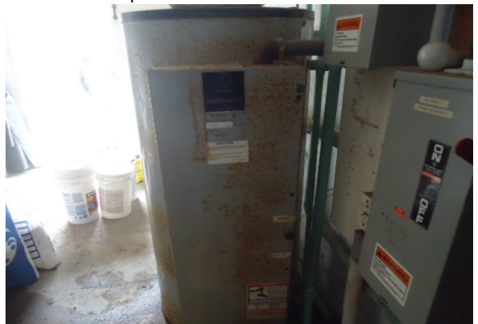
Hot water heater is beyond its expected useful life. Reserves provide funding for replacement when it ultimately fails.
