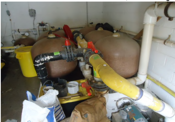
Pool filtration system that serves both pools. The main pool pump was replaced in 2021.
