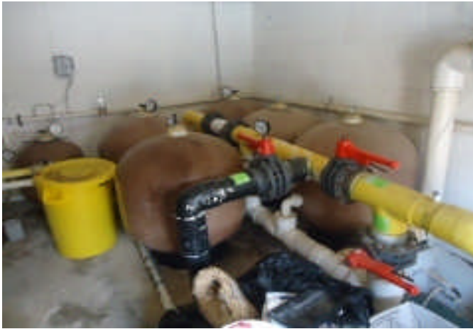
Pool filtration system that serves both pools.
