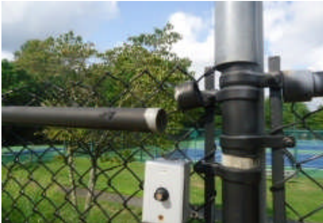
General maintenance consisting of spot repairs to rails and fence and tying up loose areas will extend the overall useful life of the fence.
