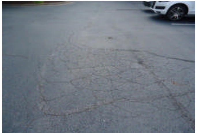
The lot is showing wearing surface and perhaps base failures. We assume the association will find it necessary to overlay the lot in about three years.
